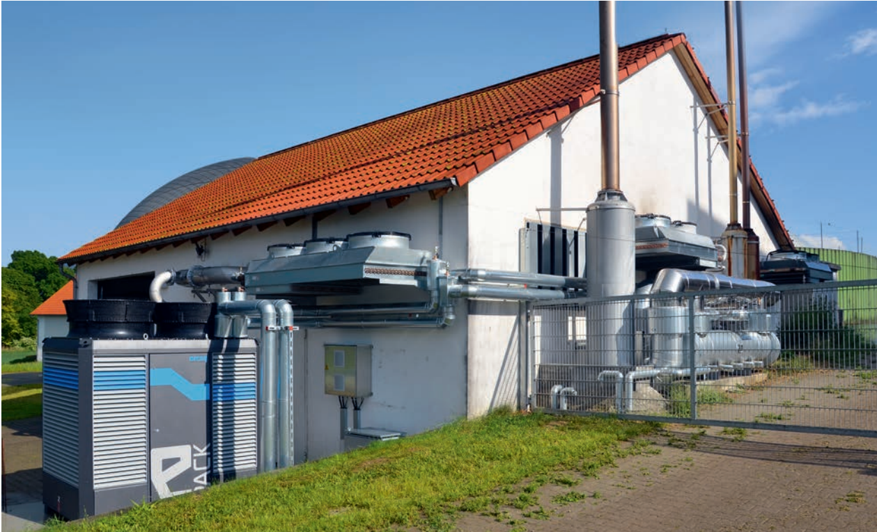
Use of Orcan Energy's compact ORC module in an anaerobic digestion plant.
