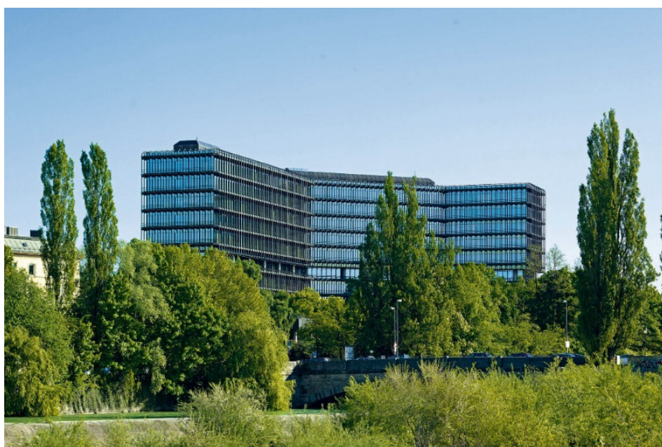
Figure 14 – OEB Munich, bâtiment Isar
