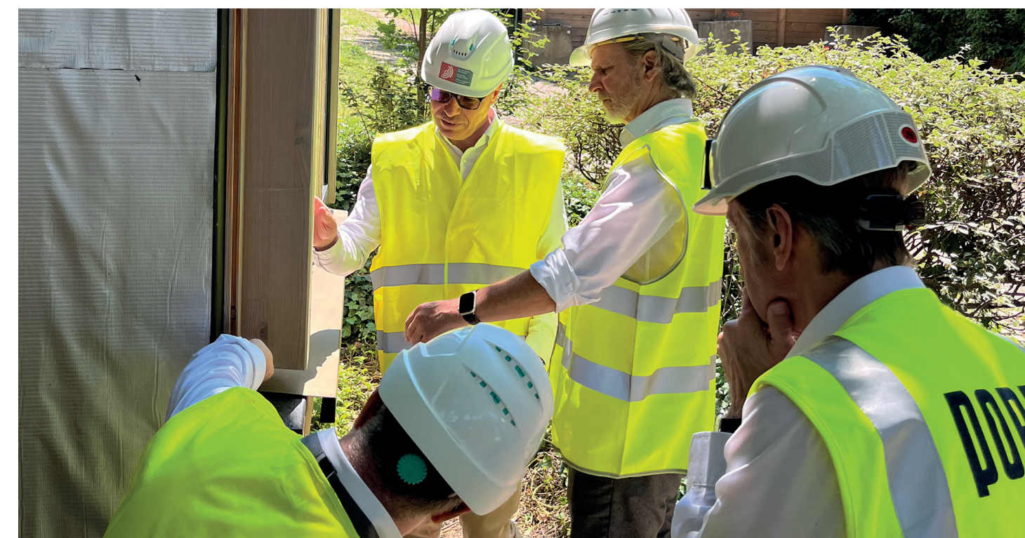
Figure 11 – Visiting the Vienna Green Hub construction site
