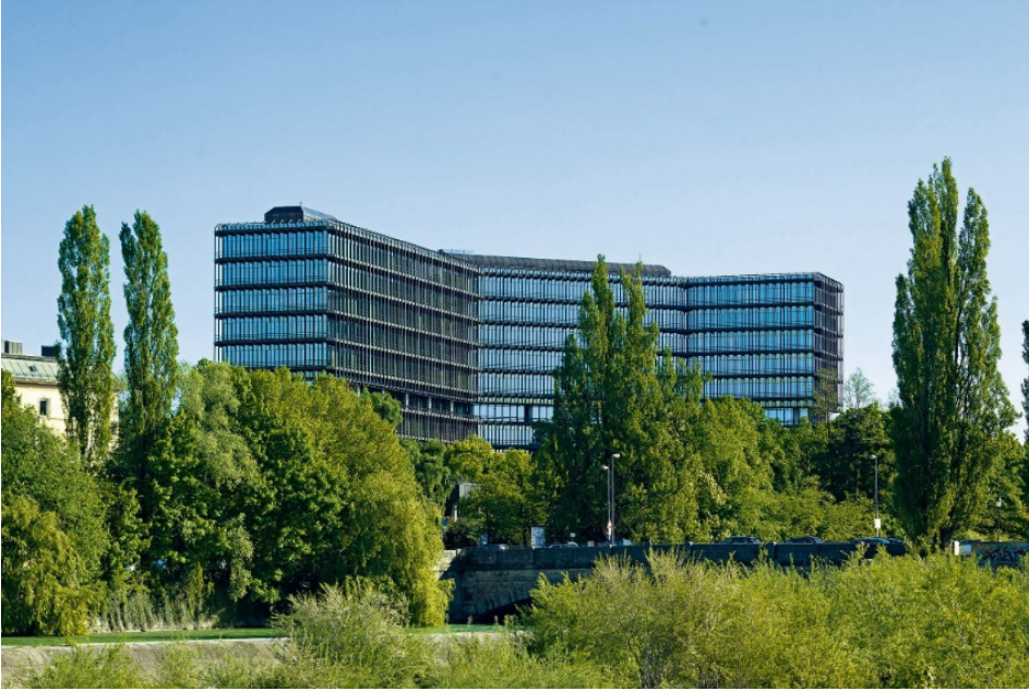
Figure 13 – OEB Munich, bâtiment Isar
