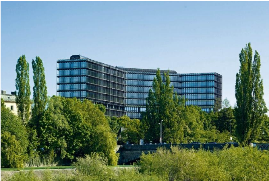
Figure 17 – EPO Munich, Isar building
