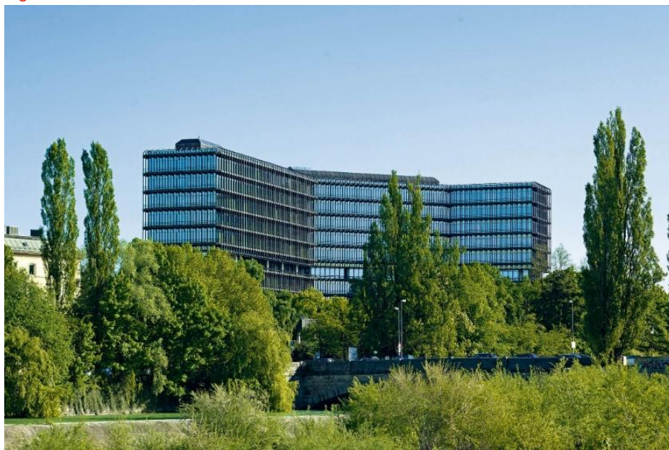
Figure 17 – OEB Munich, bâtiment Isar
